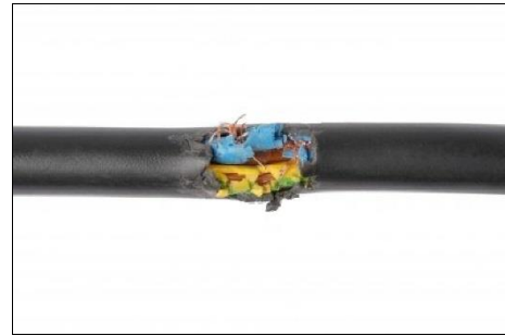
Damaged electric cable
